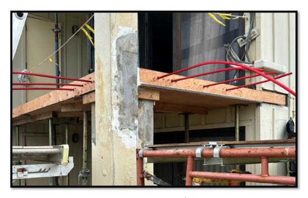
• 5 new full-length cables installed at north end of 3<sup>rd</sup> floor slab at makai side of the building
